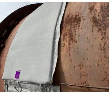
This innovative approach made the installation process quick and relatively painless for the facility, as it was completed over a weekend using only a boom lift. The modular design also makes servicing the dryer easy, as only small parts of the entire insulation jacket need to be removed to access the dryer. Additionally, putting the insulation back on is using a combination of hook and loop (i.e., Velcro®), straps, and D-rings.
